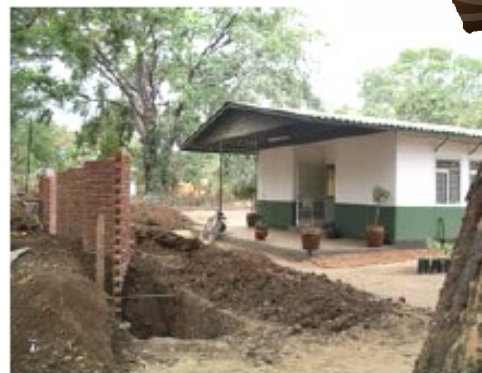
Compound Wall – Looking to the entrance of NMPCC
